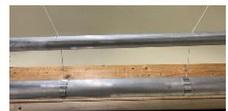
14. Starting 12" in from side of glazing bar, wrap each cord 2 times OVER TOP OF MOTOR TUBE TOWARD THE CENTER of tube. Wrap cords taut around tube but not enough to lift the bottom of shade.
