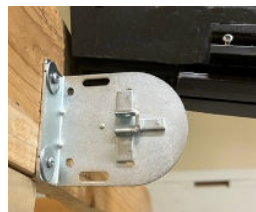
Bracket mounted to ridge wall (motor end bracket)
